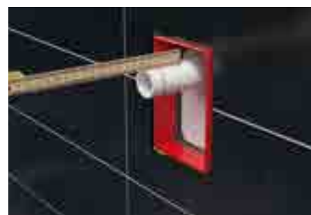
6. Mark 3cm, measured from the wall (tile)
